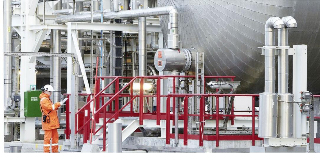
Why do ASUs explode? The most feared reason is accumulation of hydrocarbons in liquid oxygen which can take place in the main condenser unit.
