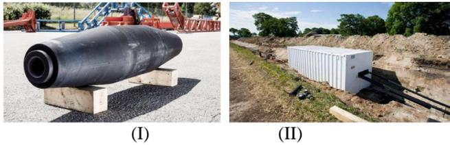
**Figure 6, (I) A 525 kV rubber body, (II) A specifically built container for underground cable jointing**
