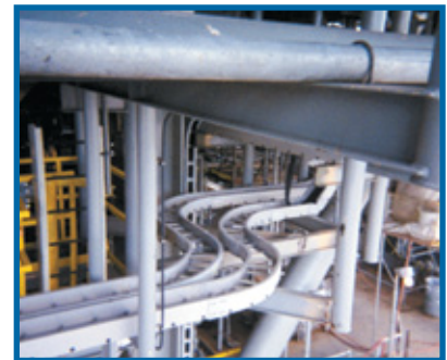
Horizontal bends change direction of tray suspended from deck above
