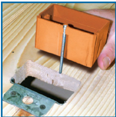
Install clip over subfloor.
