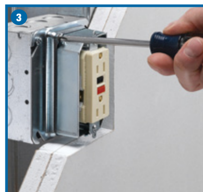
Re-tighten... Adjustment screws.
