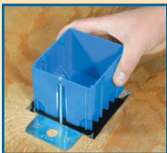
Install clip over subfloor.
