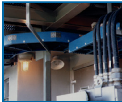
Horizontal (suspended) tray, with vertical drop to machinery below
