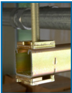
New method using Trapnut® Strut Fastener.
