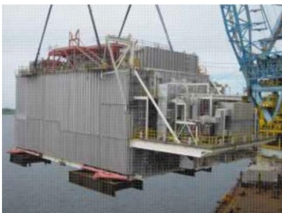
Figure 4. HVDC module lifted to platform
