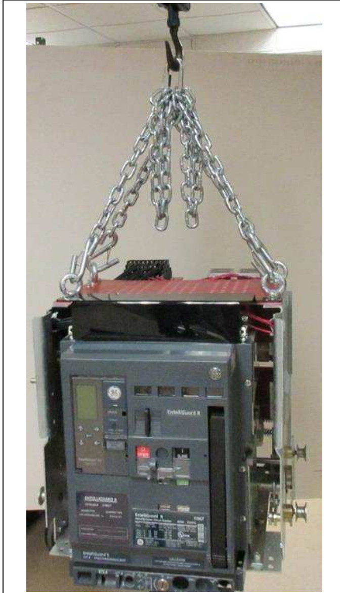
Figure 8D. AKD-10—Using eye bolts, chain and connector.
