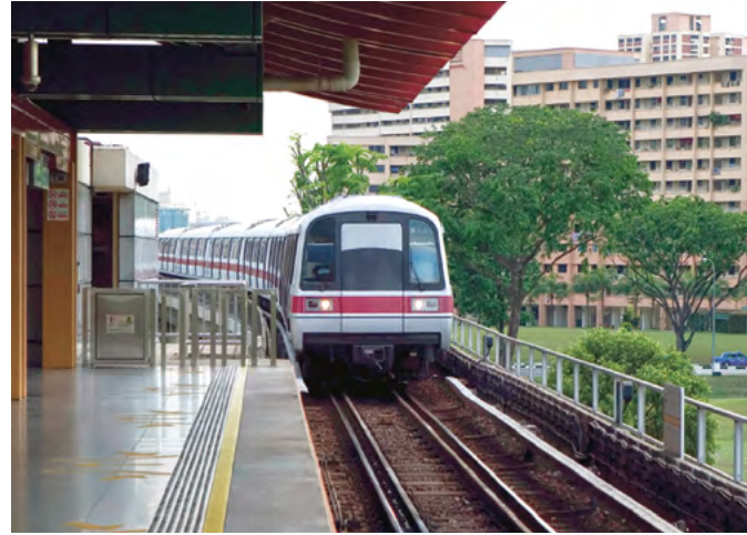
Circle Line, Mass Rapid Transit System, Singapore.
