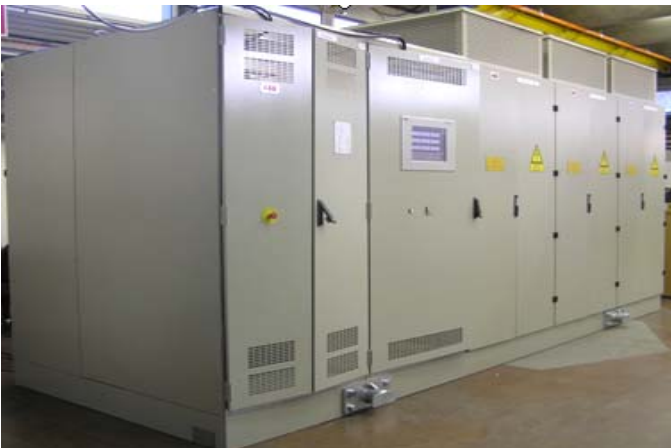
Figure 5. Cycloconverter racks with AC 800PEC controller.
