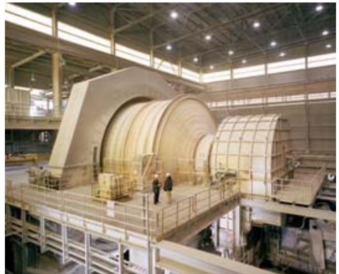
Figure 2. Ringmotor of the Gearless Mill Drive (GMD) System.
