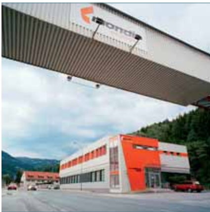
1 The 125 year old Mondi Packaging Frantschach mill sits in the Lavant Valley amid the southern Austrian Alps
