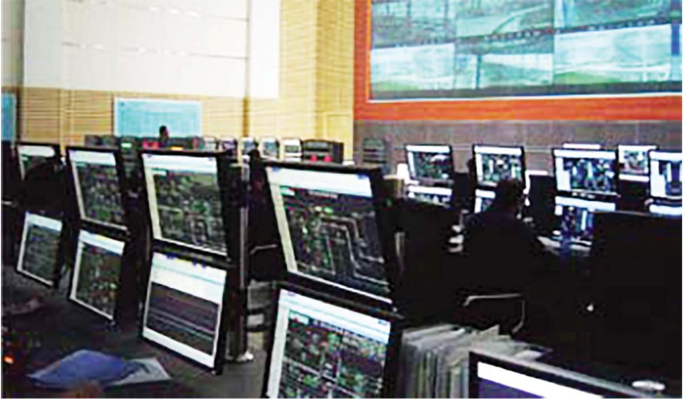
CNPS's control room
