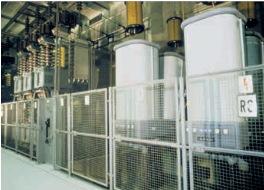
4 Mercury-arc valves and thyristor valves installed at Gotland 1
