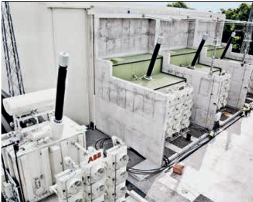
8 Converter transformers and the spare transformer at Woodland HVDC Light® station in Ireland.
