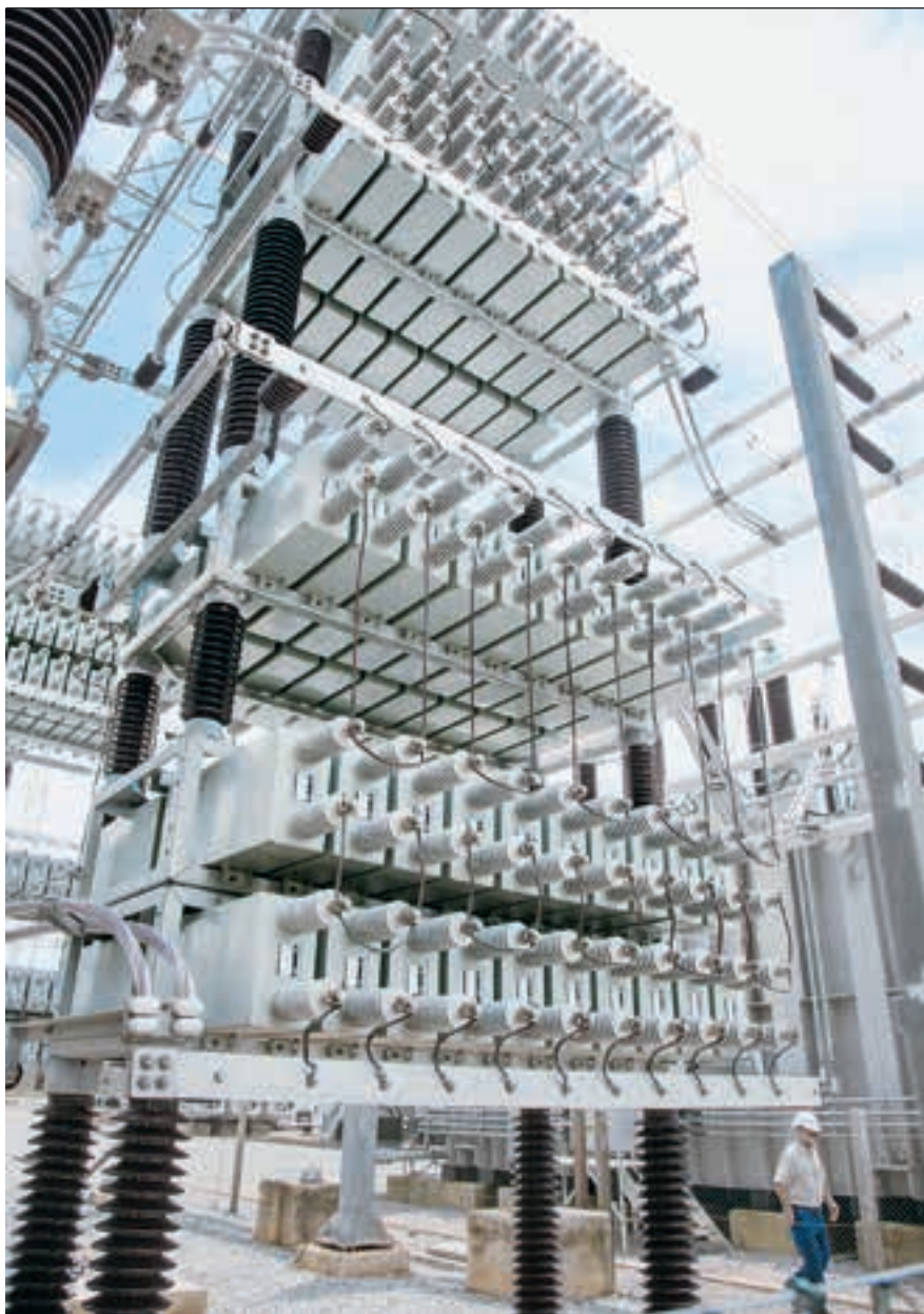
1 Capacitor bank at Porto Velho HVDC station in Brazil
