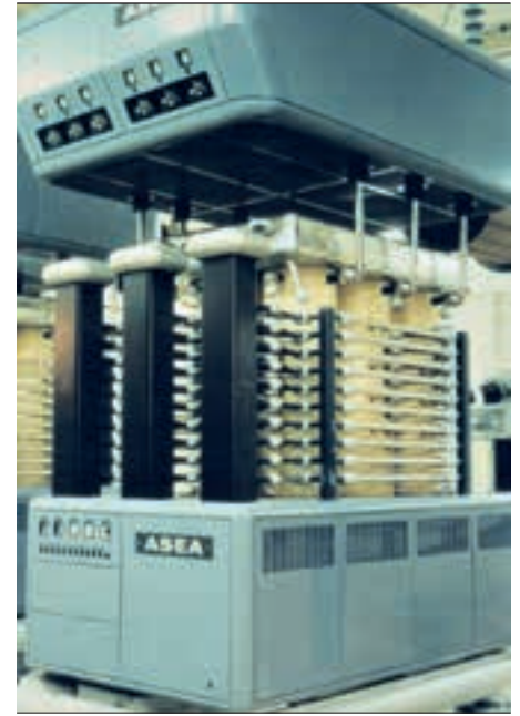
3 Pacific Intertie mercury-arc valve in Sylmar, Los Angeles
