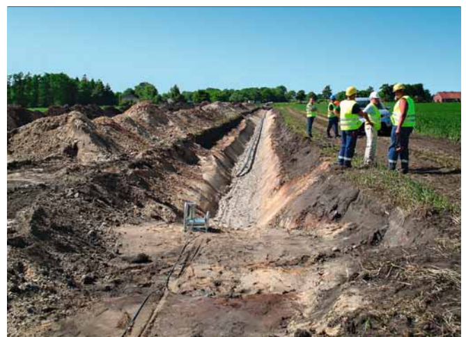
4 Laying the first sections of cable (operating voltage 150 kV, transmission rating 400 MW) in Aurich County, Germany in June 2008
