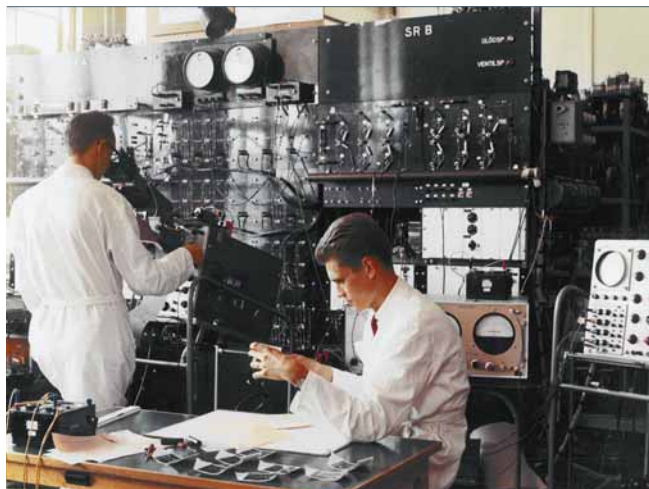
Analog simulator used in the design of the early HVDC transmission systems
