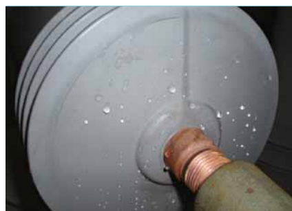
2 Water beading on the vertical surface of the HCEP cast OVR after two years in Kitty Hawk, North Carolina (Courtesy of Dominion Virginia Power).
