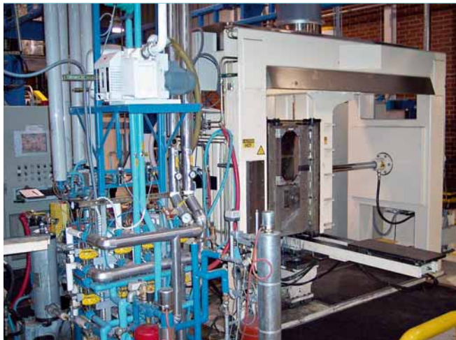
5 Automatic pressure gelation (APG) press in ABB's Pinetops facility in North Carolina.
