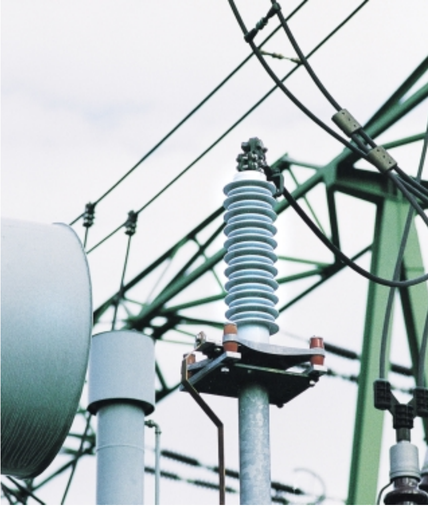
POLIM-H surge arrester with a continuous voltage rating of 44 kV, used as transformer protection in a switchyard in Switzerland
