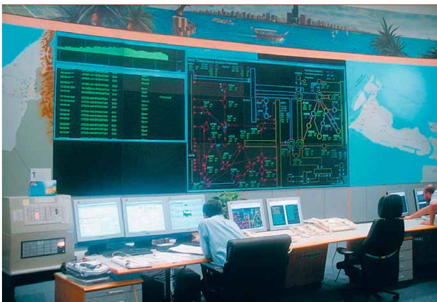
A typical control room
