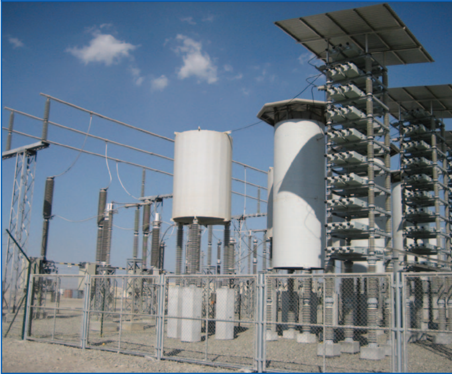
Figure 7: High Voltage compensation system
