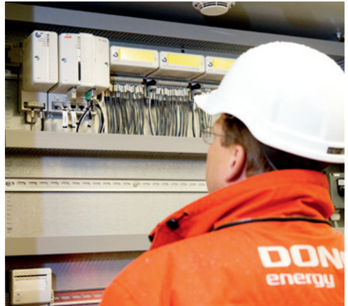
One of the eight AC 800M HI controllers with I/O modules used in the Dong Nybro gas treatment plant as part of the ESD system.
