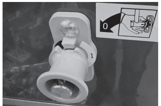
28 Check if the arrestor ring and switch-disconnector are in locking position
