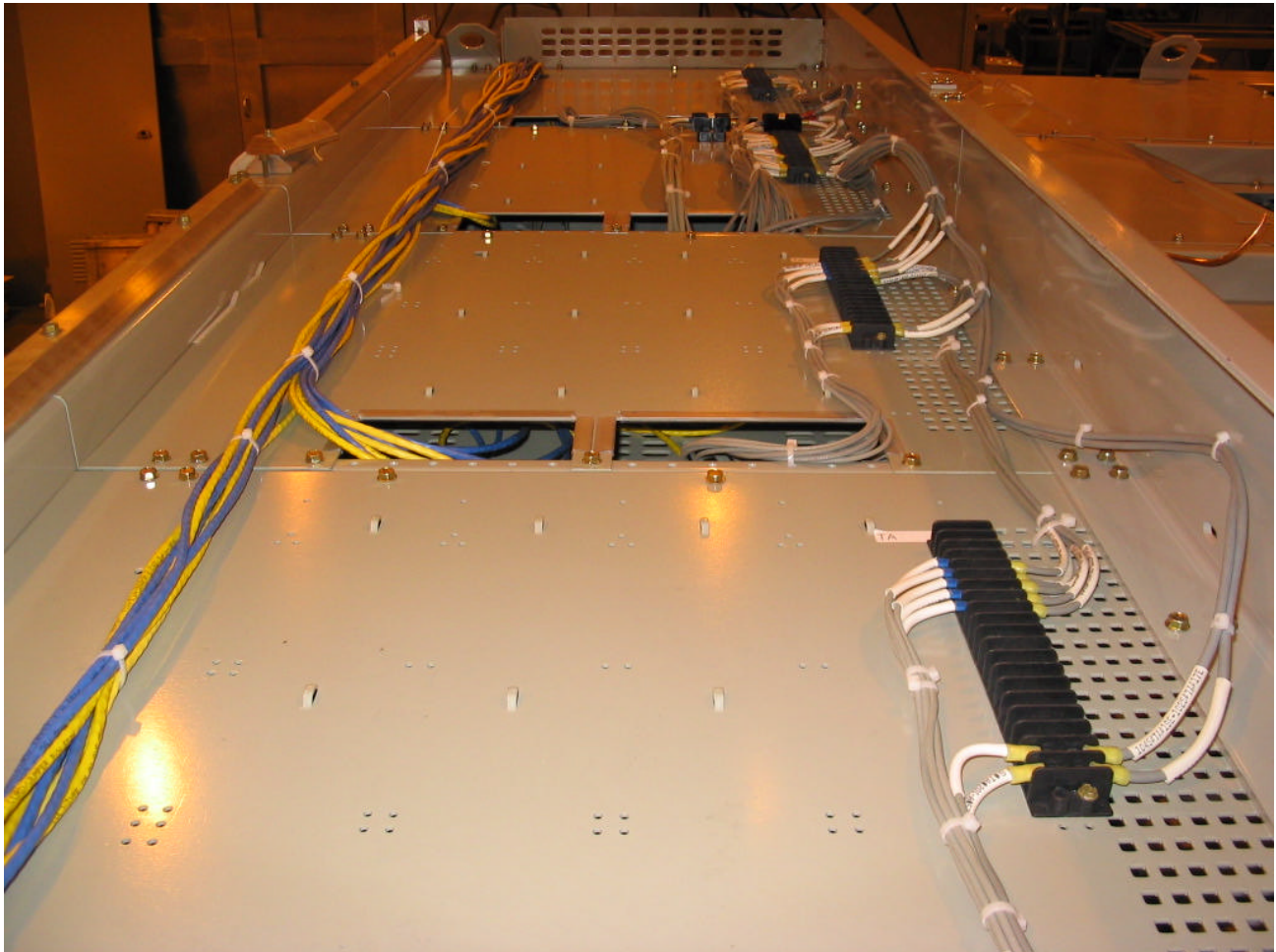
Fig. 4-14. Interconnect control wiring and Ethernet cables in the wiring trough on top of the equipment
