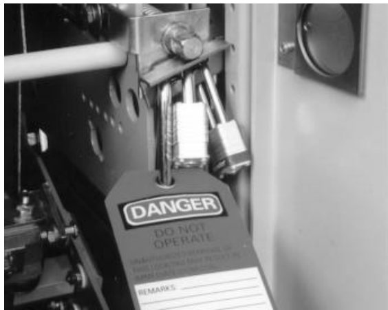
Fig. 7-7. Racking mechanism padlock device (EGS-32/40/50 breakers)
