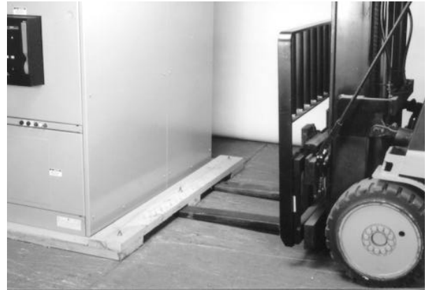
Fig. 2-4. Placing forklift tines under Entellisys equipment shipping skid
