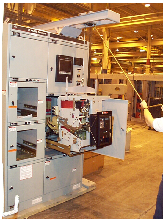
Fig. 5-6. Pull rails out completely from the circuit breaker compartment
