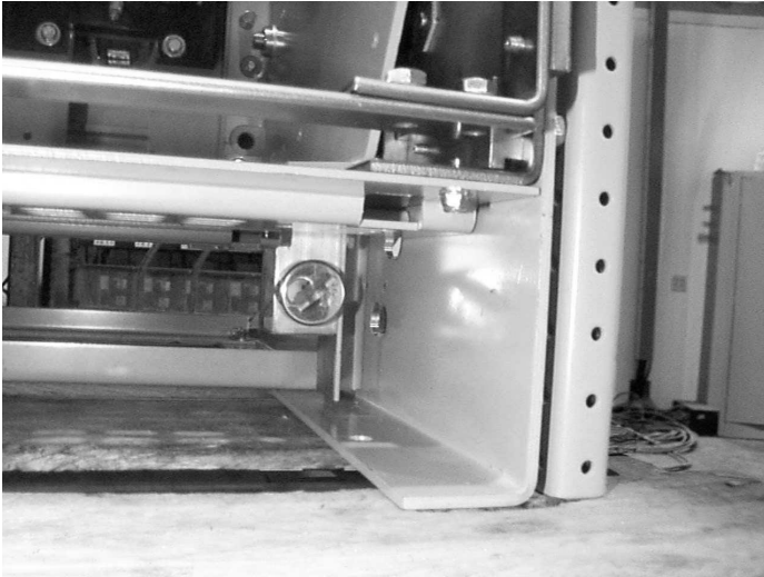
Fig. 5-19. View showing FRE key interlock locking FRE in connect position
