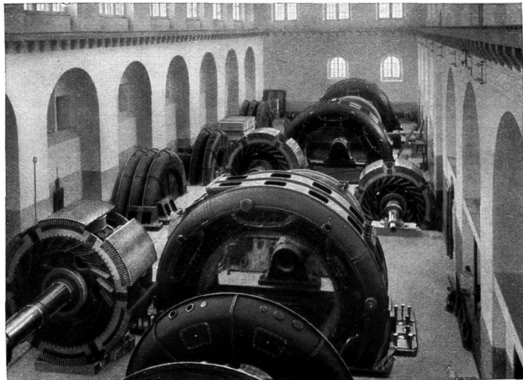
Fig. 4. — General view of the first three alternators in course of erection.
