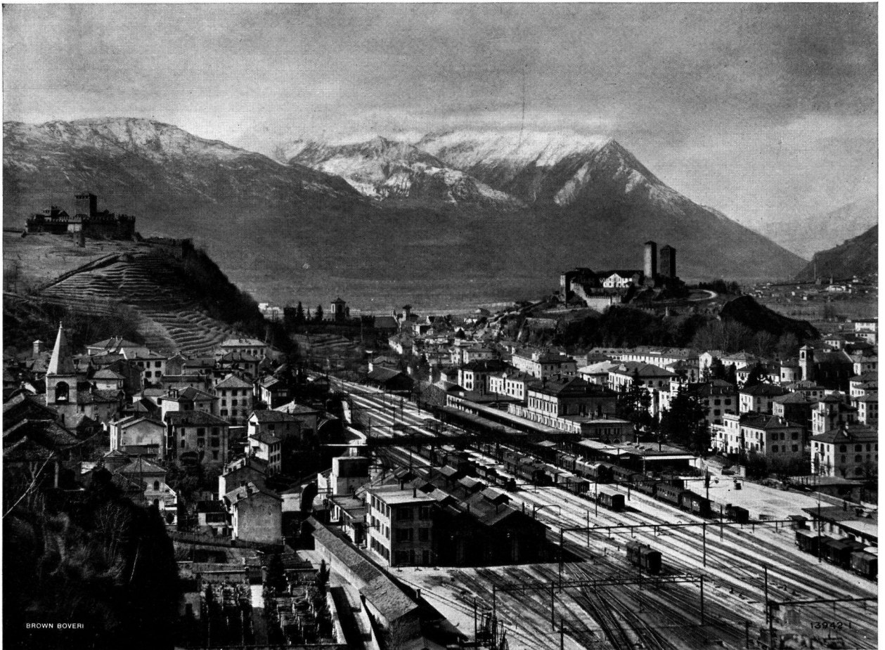
BELLINZONA STATION OF THE ELECTRIFIED LUCERNE-CHIASO SECTION OF THE GOTHARD RAILWAY.
