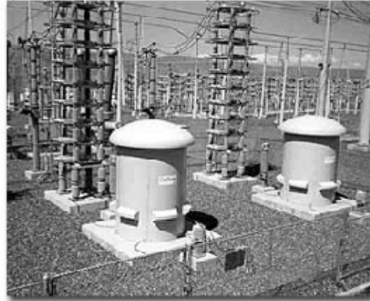
Fig. 3 ConTune filter installed in the Celilo station of the Pacific Intertie HVDC transmission
