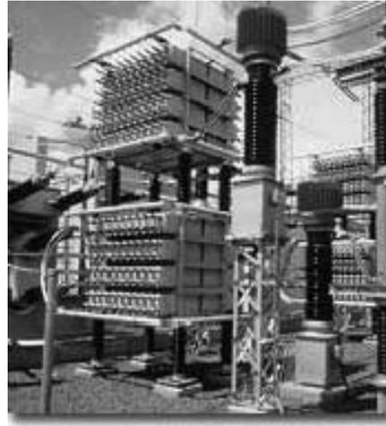
Fig. 6 Commutation capacitors at Garabi.
