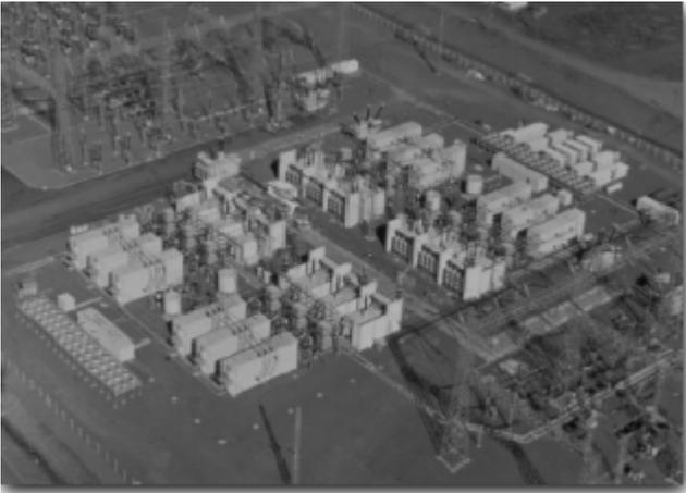
Fig. 7 Overview over the central part of stage 1 of the Garabi 2\*550 MW back-to-back station.
