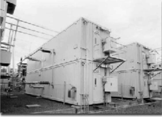
Fig. 1 The outdoor HVDC valves at Garabi are placed on top of each other to save space.
