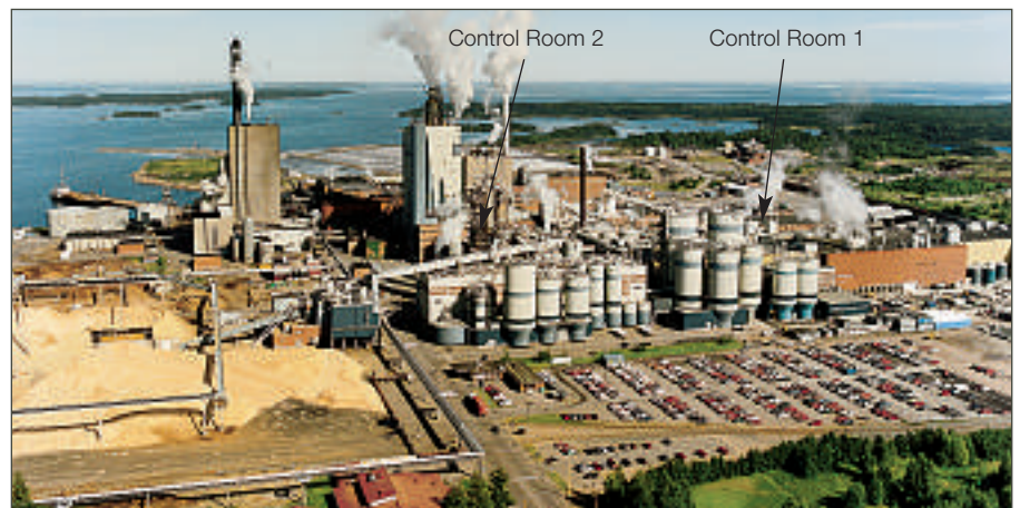
Korsnas paper mill. The site, which previously had 13 control rooms, now only has two. ABB's integrated automation solutions make this possible.
