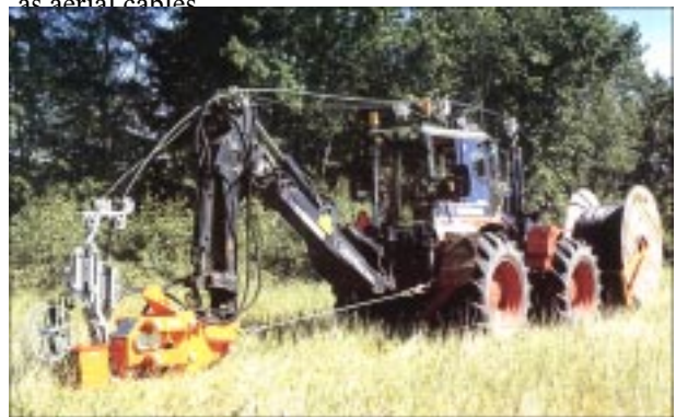
Fig 3. shows cable ploughing technique
