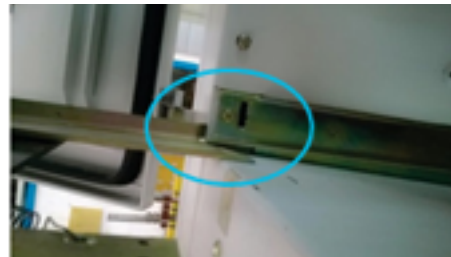
Figure 5-11. Lift Truck Arm (Left) Aligned with Switchgear Guide Slot (Right)
