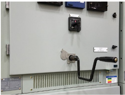
Figure 5-26. Racking Handle
