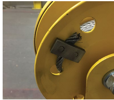
Figure 5-10. Cable Secured to Hoist
