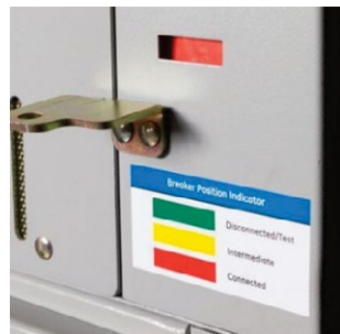
Figure 5-31. Connected Position (Red)
