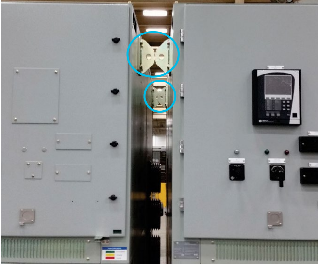
Figure 4-4: Lift Plugs in Position
