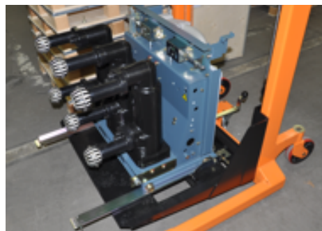
Figure 5-6. SecoVac VCB Properly Mounted on Lift Truck
