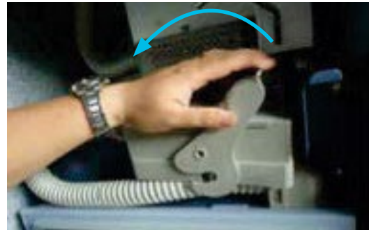
Figure 5-24. Release Secondary Plug from VCB
