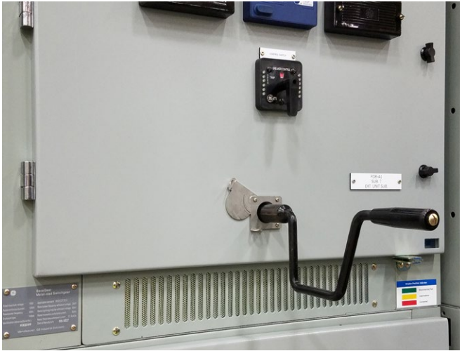
Figure 3-2: Circuit Breaker Manual Rack in/out
