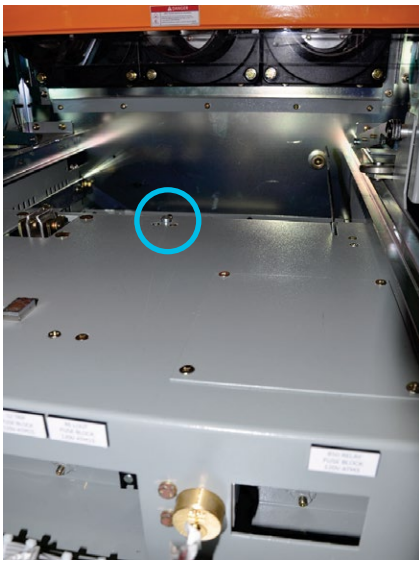
Figure 9-12: Initial Stopper Rod Position
