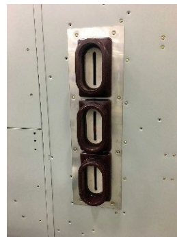
Figure 4-19: Side Bus Shrouds
