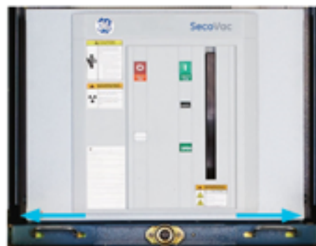
Figure 5-18. Lock VCB into Switchgear
