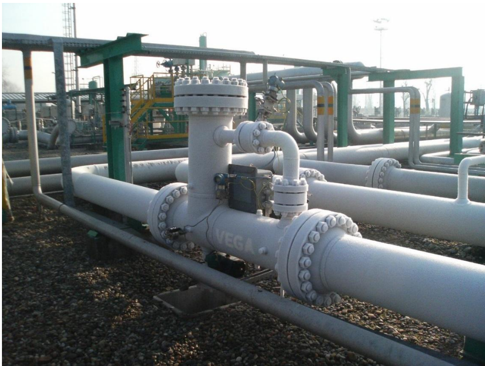
Figure 7 – Isokinetic Sampling-based MPFM installation in Ripalta
