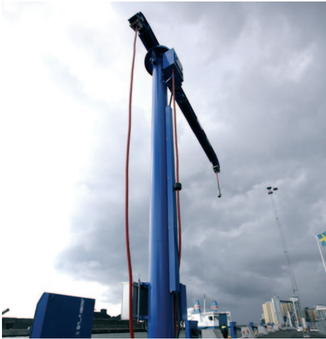
One of the cranes enabling the shore-to-ship connection
