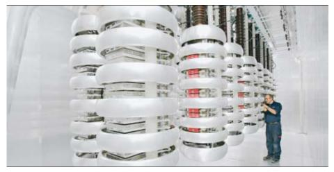
The characteristic, above all others, that makes HVDC Light so controllable is mainly due to the IGBT semiconductor devices used in its assembly. Like thyristors, IGBTs can be connected in series to increase the voltage ratings.
