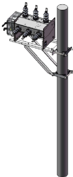
Single pole installation
