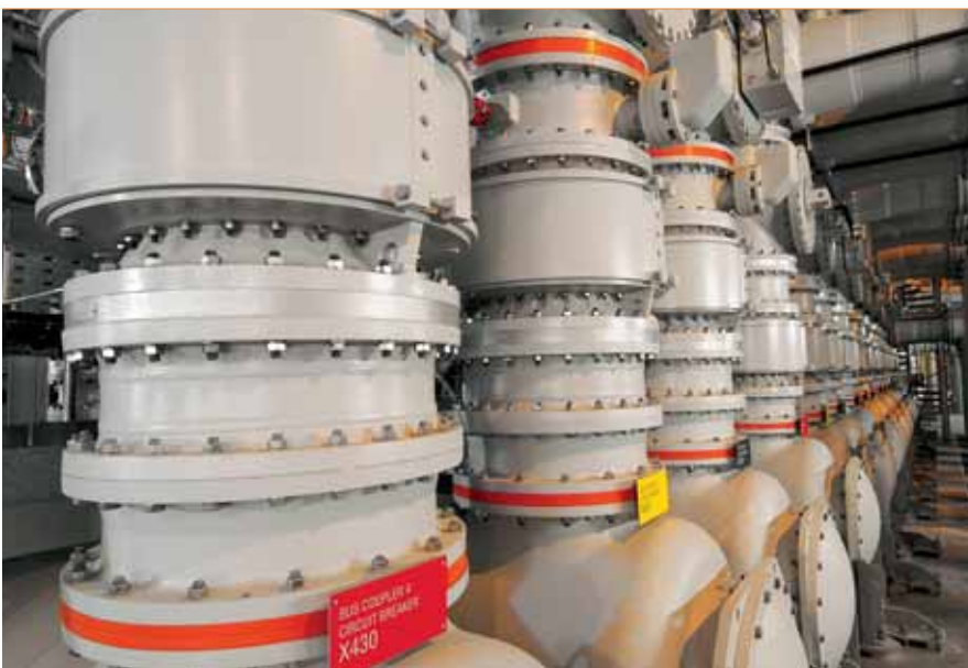
3 ABB's compact gas insulated switchgear has the right footprint.
