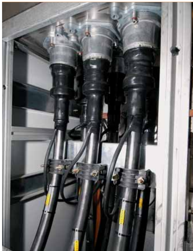
1 ABB 400-kV XLPE underground cable
