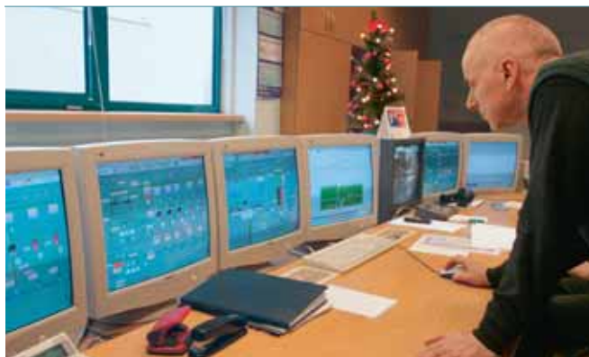
4 The control system is based on ABB’s Advant architecture
