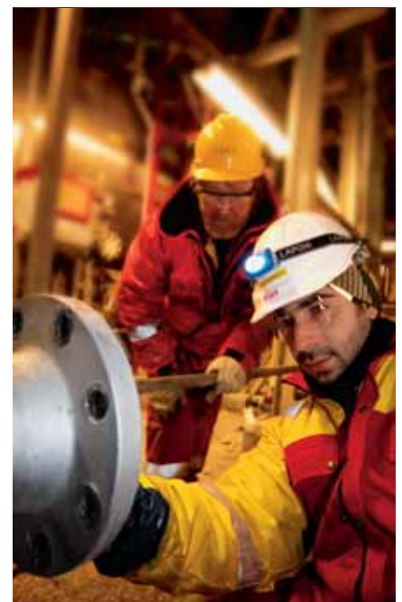
Men at work on the Snøhvit installation [Photo: Marit Hommedal/Statoil]
