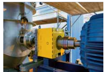
4 The pump that keeps the water flowing is powered by an ABB frequency converter
