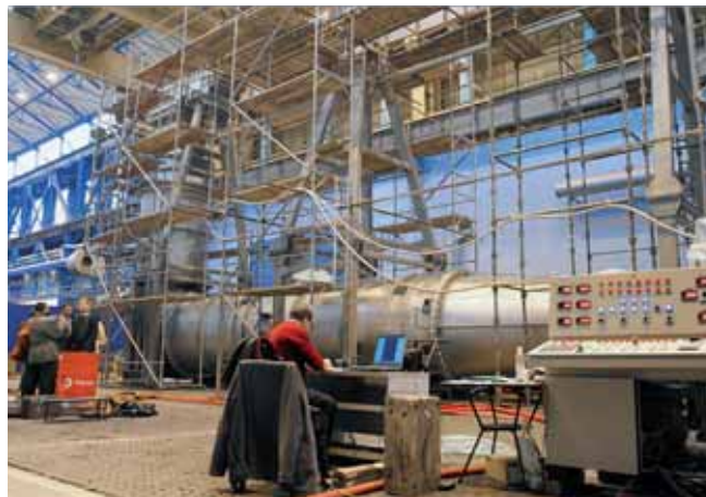
6 Numerous tests were required to verify and ascertain the tunnel’s properties
