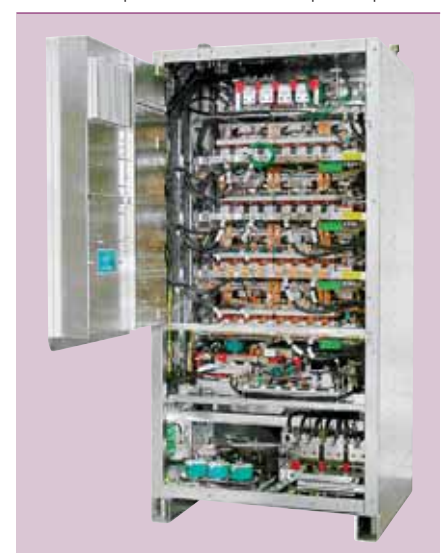
3 The control hardware of the CC750® swivels aside to permit access to the power part
