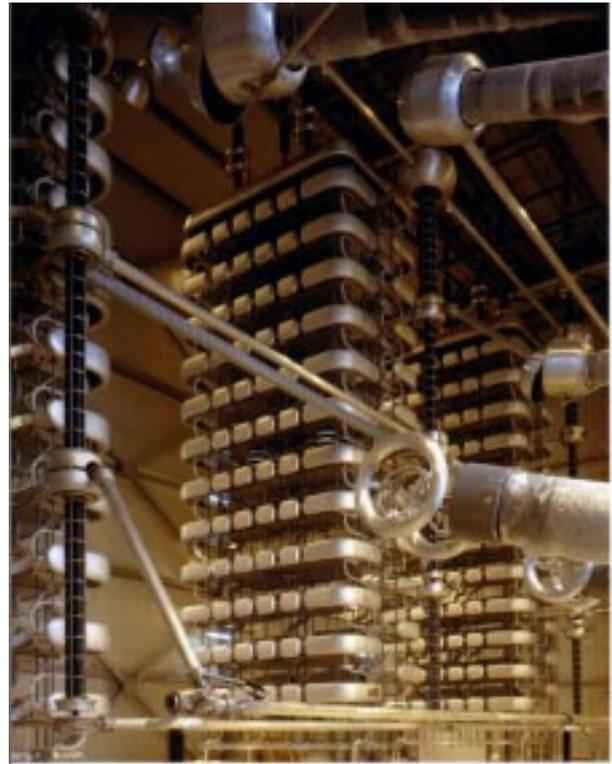
Fig.7 – Thyristor bridge structure.
