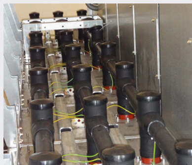
Busbar compartment with support for voltage transformers
