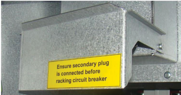
Fig 11: Secondary plug and arrangement photo.
