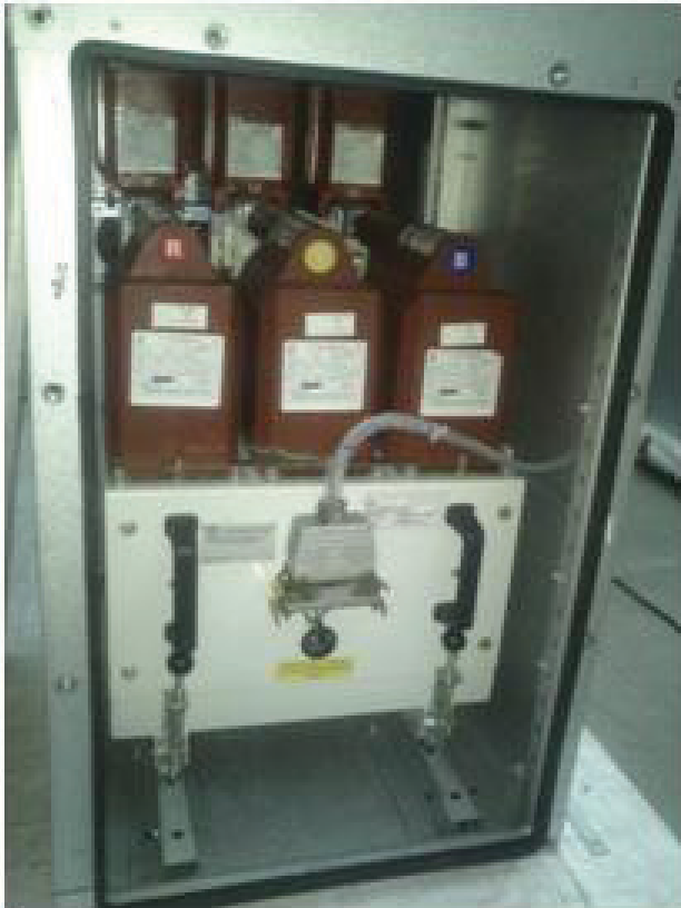
Fig 50: Withdrawable voltage transformer
