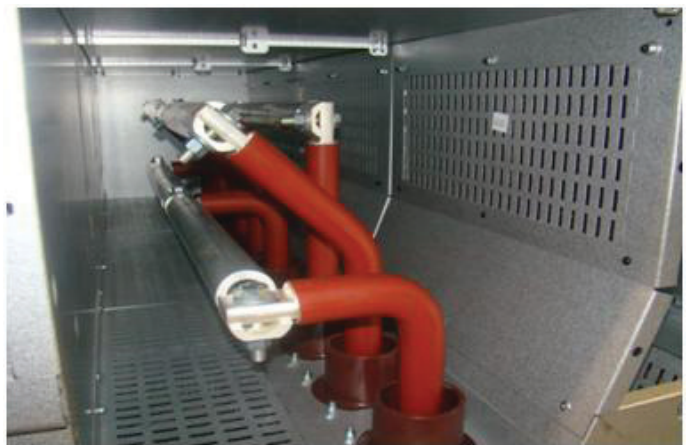
Fig. 35: Busbar assembly.
