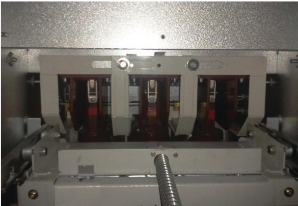
Fig.23: Circuit-breaker compartment, open withdrawable part in service position
