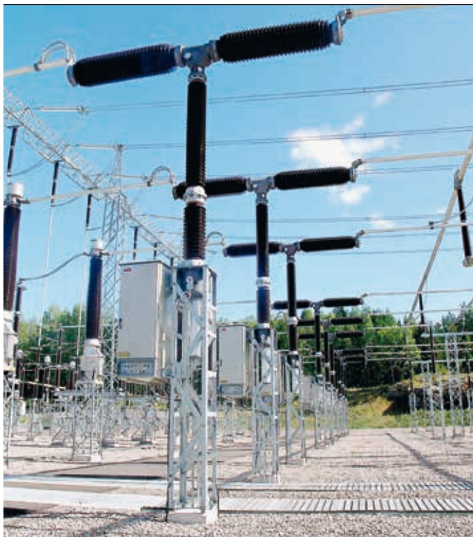
4 Modern 420 kV SF 6 circuit breaker with two interrupting units in series
