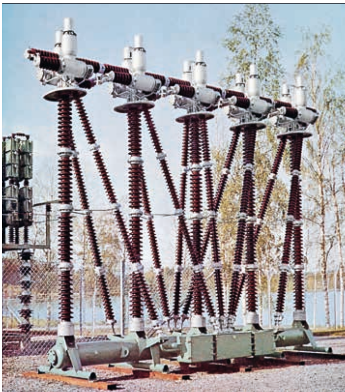
3 420 kV circuit breaker airblast technology from 1955 with 10 interrupting units in series
