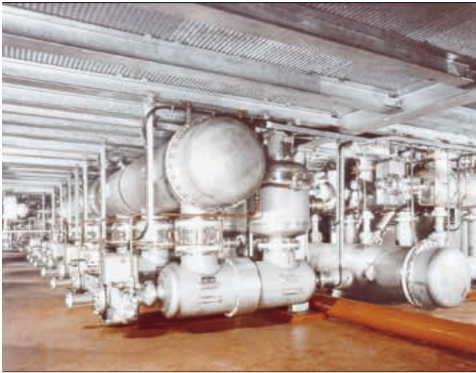
1 Gas-insulated switchgear (GIS), Sempersteig, Zurich, 1967
