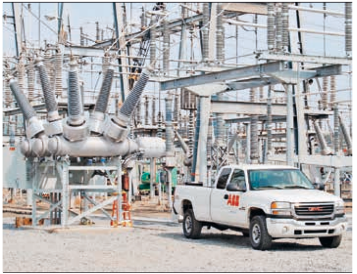
2 Dead tank breaker, United States
