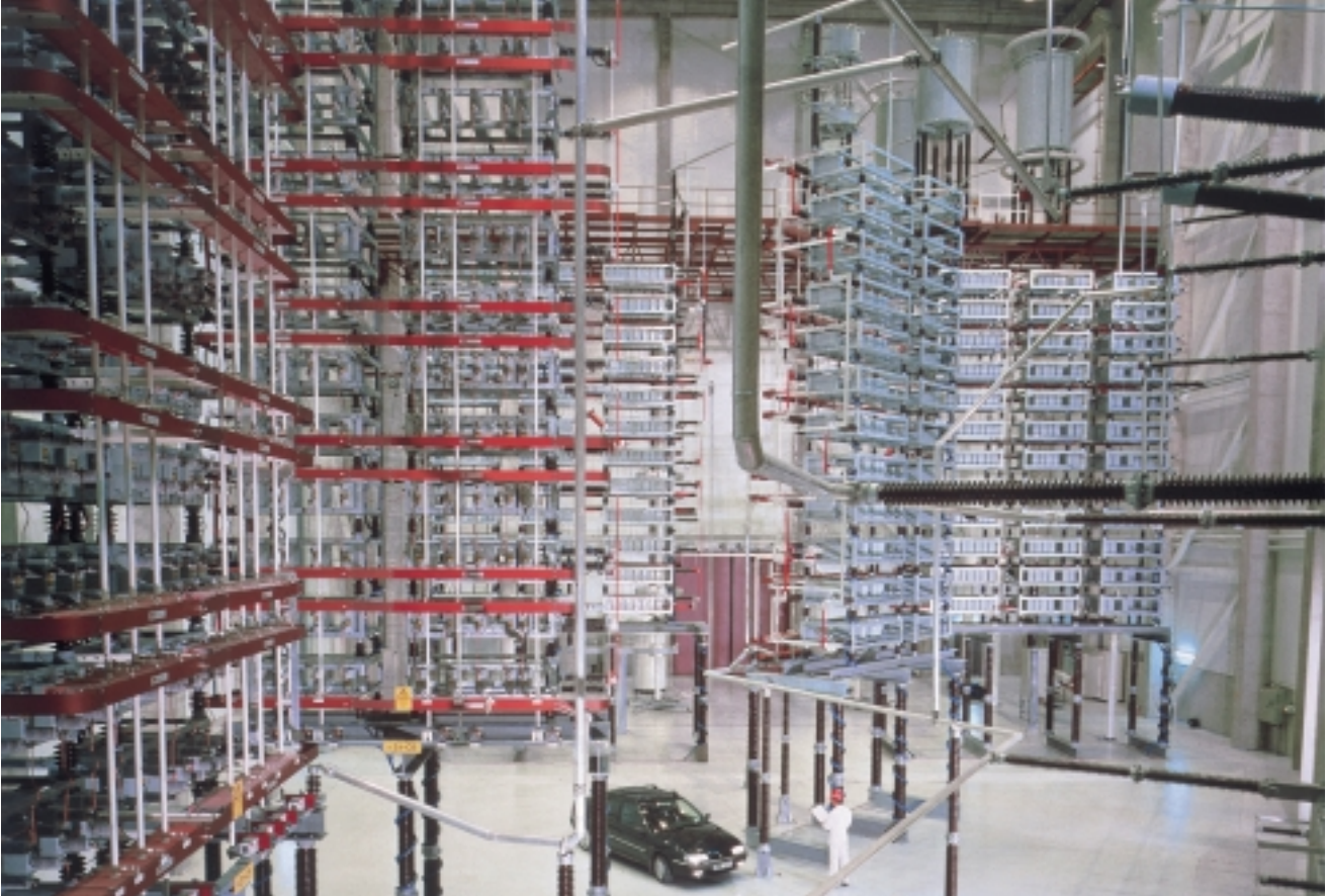
View inside the building with the voltage circuit. The bay is 30 m wide, 60 m long and 30 m high.
