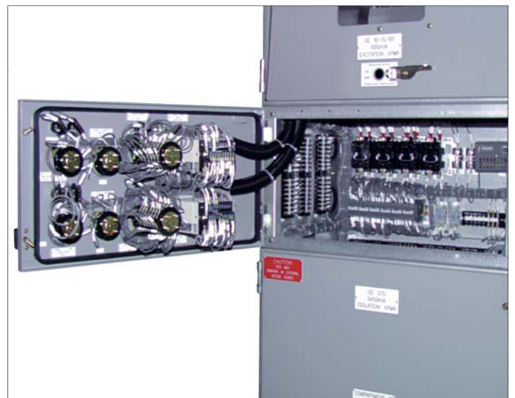
Low voltage instrument module isolated for maximum safety when working with low voltage circuits
