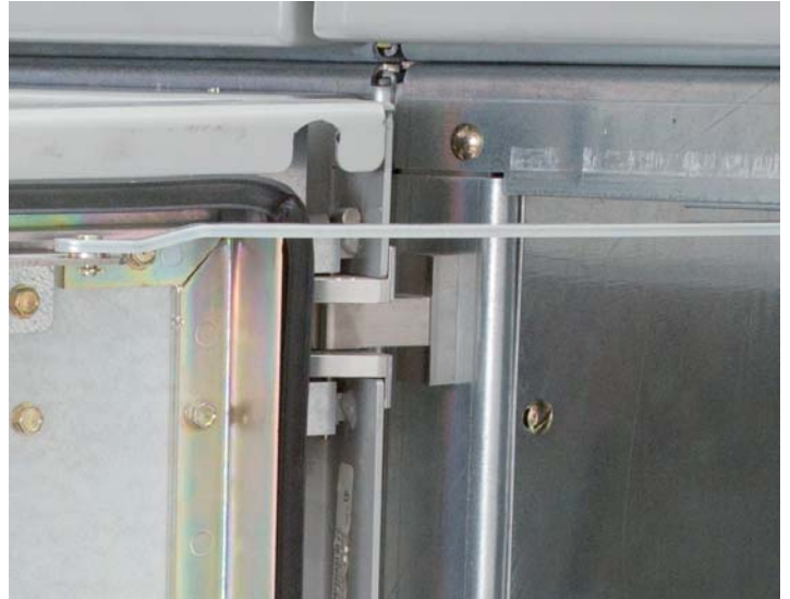
Hem bending creates a rigid structure and sturdy construction in arc resistant metal-clad switchgear (reinforced, arc resistant door construction shown).
