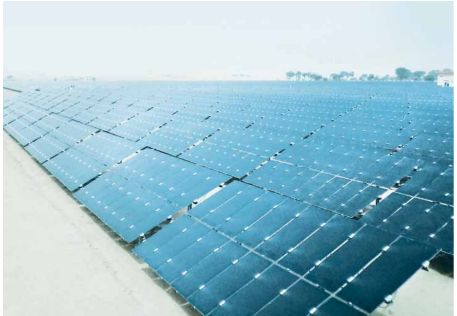
Punj Lloyd solar plant site at Bap, Rajasthan
