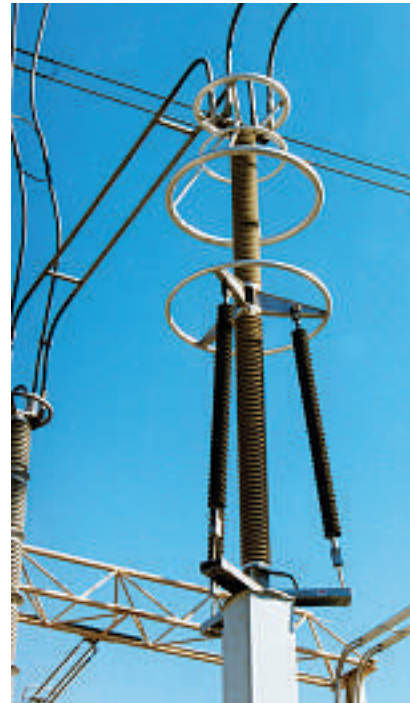
3 Earthquake-resistant surge arrester with polymer housing
