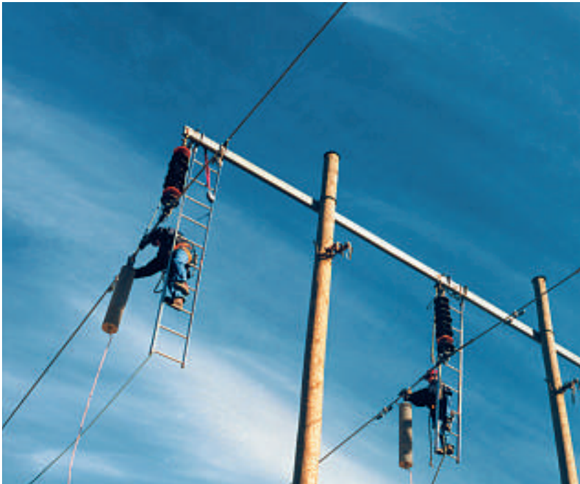
2 Installing polymer-housed surge arresters on a transmission line – now a safer and simpler task
