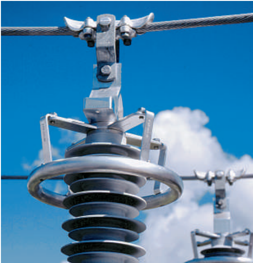
6 PEXLIM arresters installed on transmission lines in a 400-kV grid. The hollow insulator is also made of polymer.
