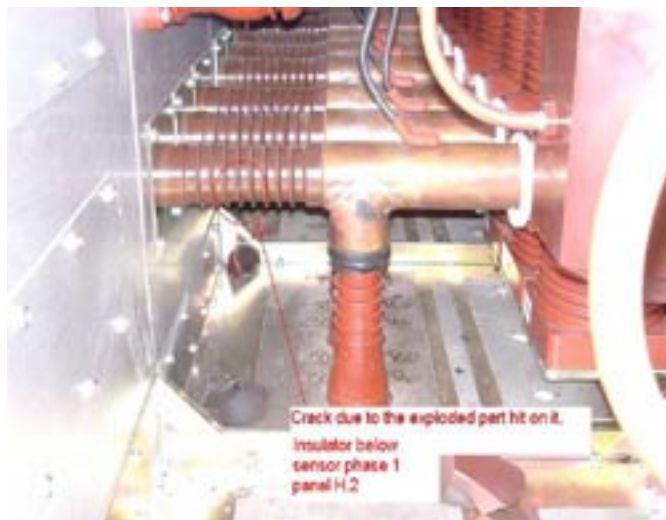
Fig.1 Open arc failure, with Arc Eliminator
