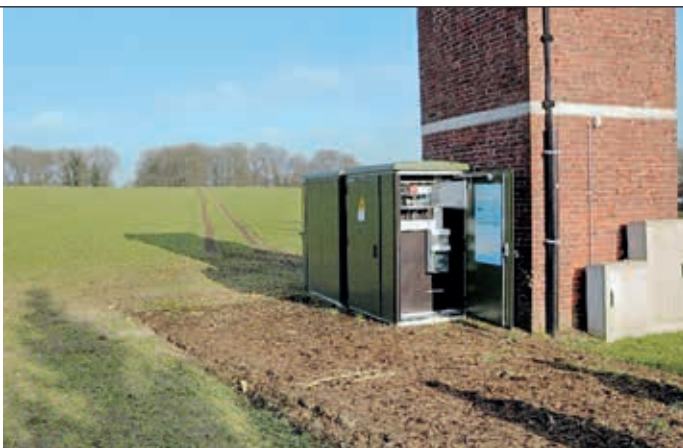
4b Dedicated cabinet solution containing new switchgear and "intelligence" added to existing substation
