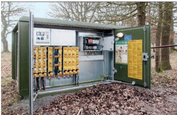
4a New intelligent compact substation
