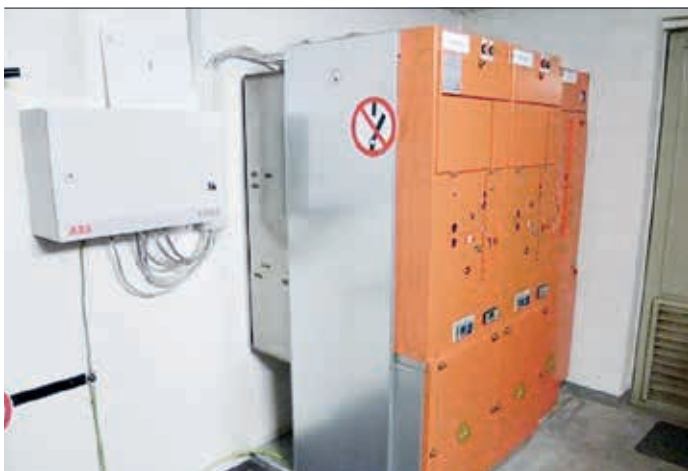
4c Replacement of existing switchgear in a walk-in substation
