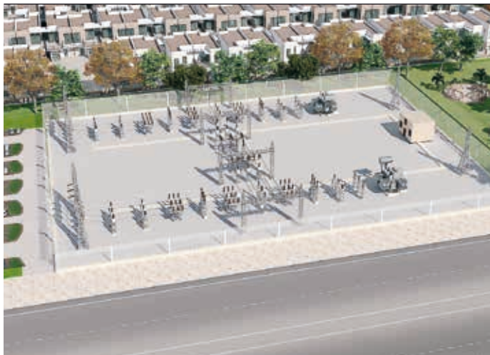
4a Air-insulated switchgear
