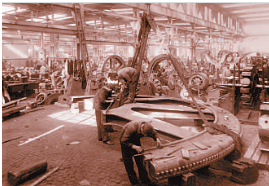
Generator assembly in Baden, Switzerland, 1895
