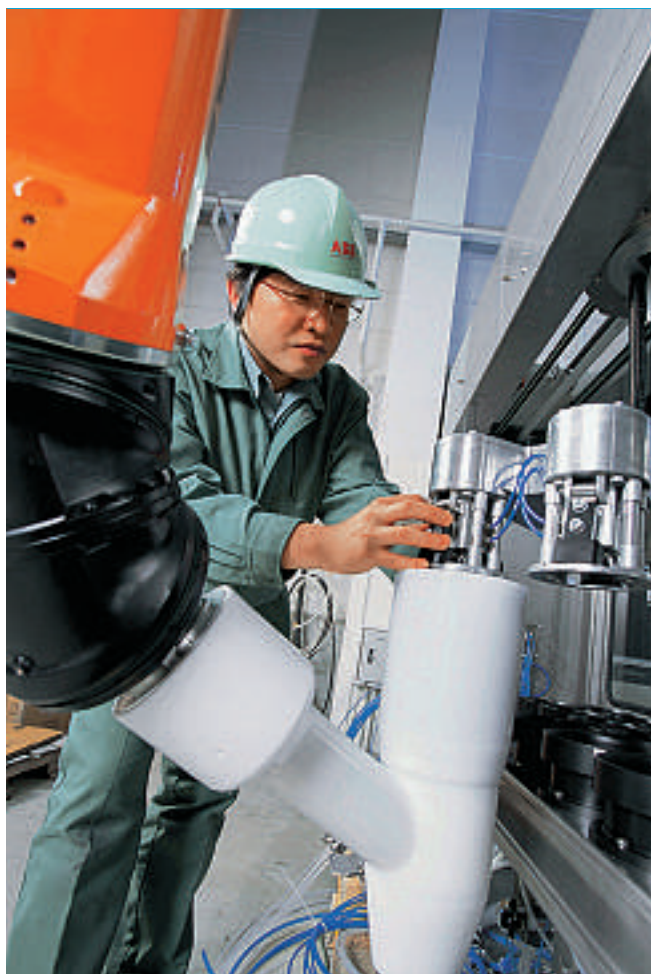
3 An ABB technician inspects a CBS installation
