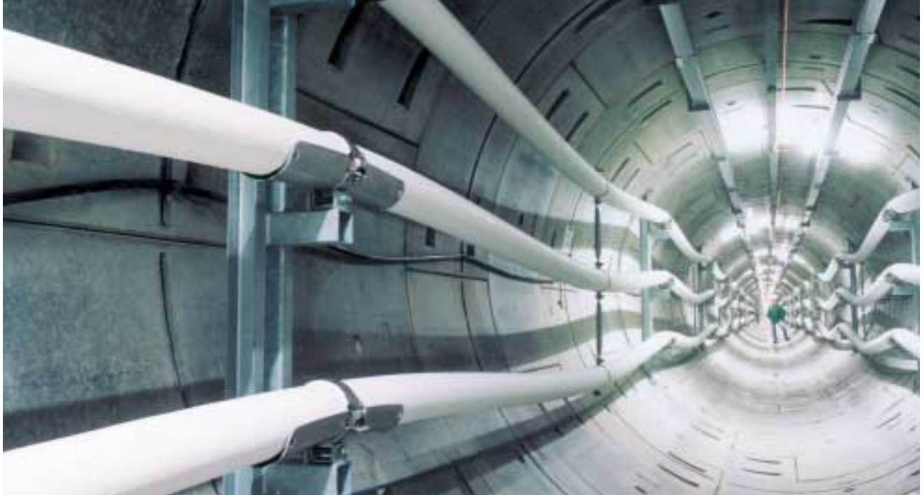
8 400-kV cable system in a 6.3 km underground tunnel running through Berlin's city center
