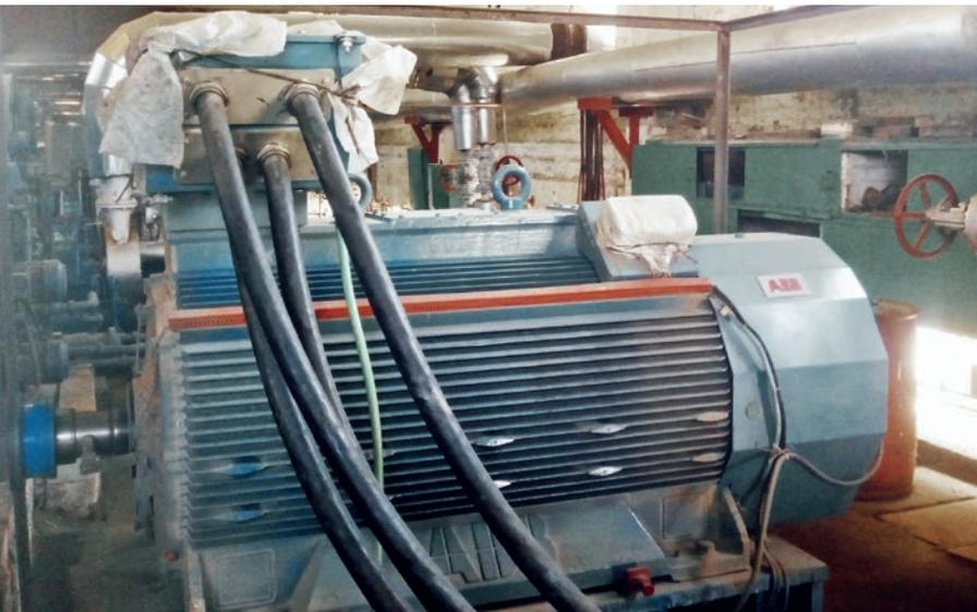
Switching from an old-fashioned steam turbine to a modern ABB rib cooled motor and drive package on its cane crusher helped Mirpurkhas Sugar Mills in Pakistan to reduce energy use by more than 40 percent.
