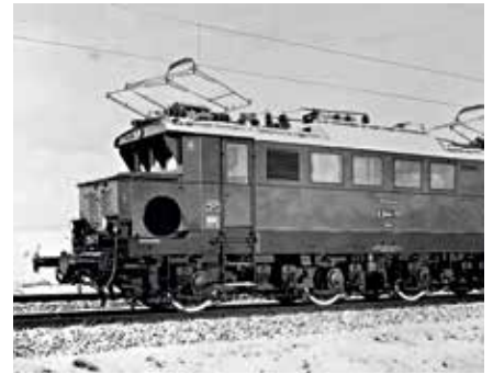
1938 First locomotive using multianode mercury-arc rectifiers from BBC Mannheim, Germany
