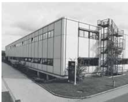
1981 Inauguration of BBC high power semiconductor factory in Lenzburg, Switzerland
