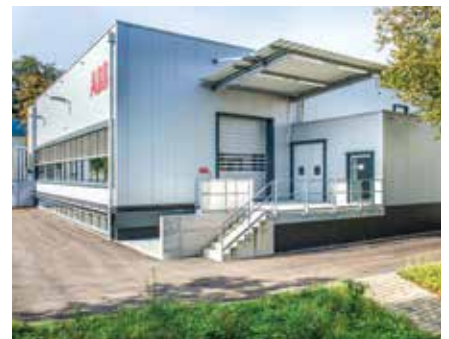
2014 Inauguration of ABB's new power electronics advanced research lab in Dättwil, Switzerland
