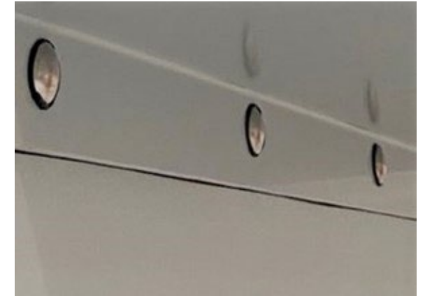
Use of self-sealing bolts in all external bolts
