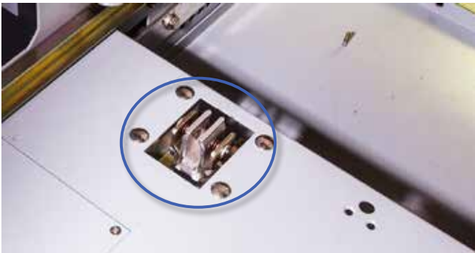
Figure 6-2: Ground Shoe in Breaker Cell
