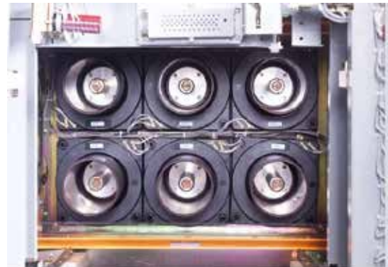
Figure 6-17: CT Mounting in Breaker Compartment
