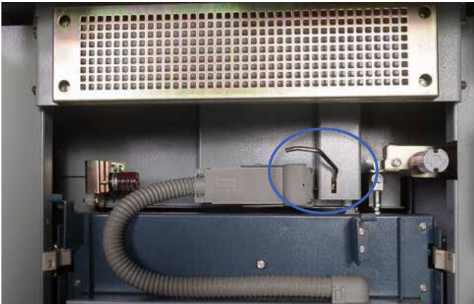
Figure 6-10: Disconnect Plug Mechanically Interlocked
