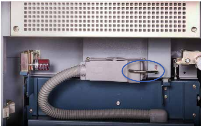
Figure 6-10: Disconnect Plug Mechanically Interlocked
