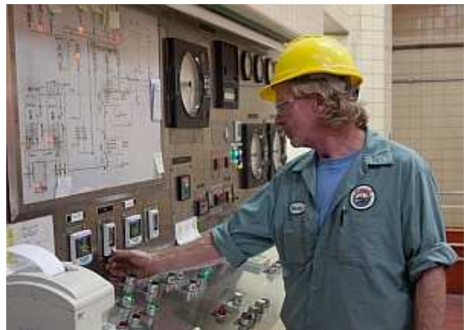
Figure 3 Operator dials wort volume of kettle in CM10 prior to wort boiling operation.
