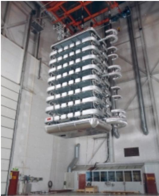
Fig.1 View of 3G HVDC thyristor valve
