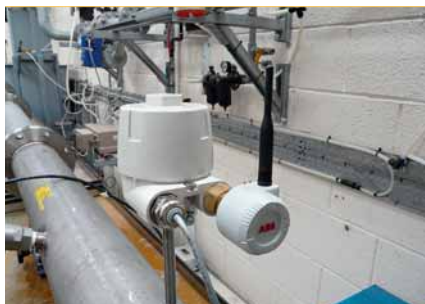
Adapter installed on-site
