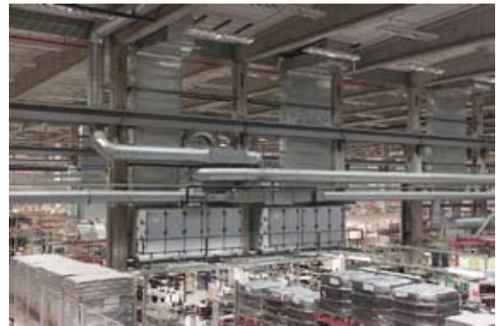
Air handling units (AHUs) and the duct work in a factory.
