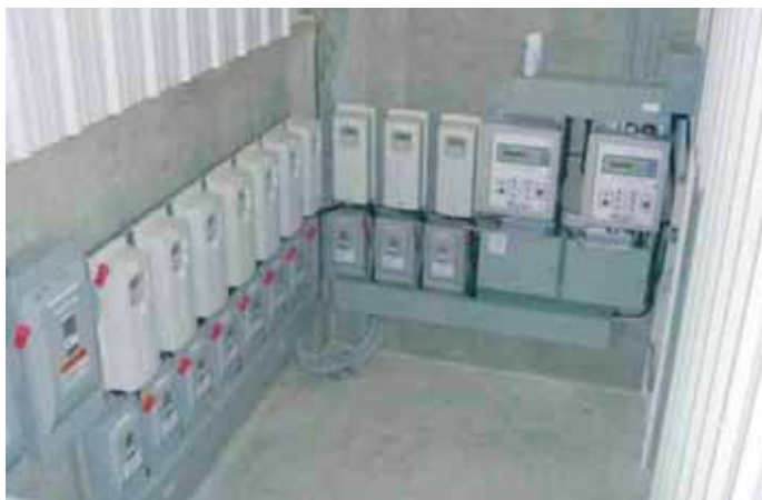
The ABB drives control the storage facilities from an electrical control room.
