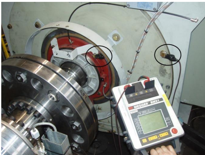
Figure 31 Measuring the insulation resistance of an anti-friction bearing
